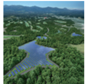
Artist’s Rendition of the Completed Nasu Shirakawa Mega Solar* Power Plant *Tentative name
